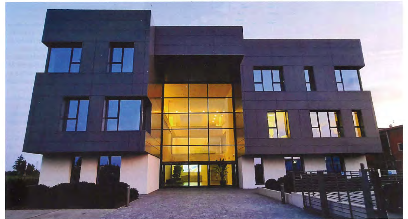
Above: IMAL's new office building at the headquarters in Modena
