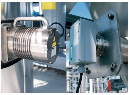
The APX300 system has been designed to prevent cyclone plugging which is one of the major causes of production downtimes.
