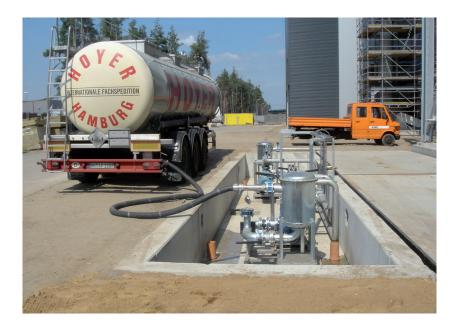
The preparation and storage systems for chemical additives such as hardener, hexa, emulsion and melted wax etc. are constructed ad hoc to meet the specific requirements of the production process, in a flexible and reliable manner with automatic computerized controls.
