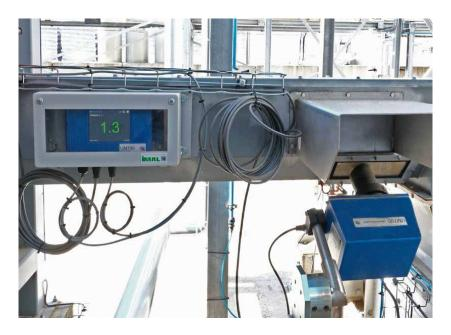
The UM700 is an infrared photometric analyser which uses fixed near infrared wavelengths to measure the amount of moisture contained in a variety of products. The system is based on the capacity of the materials to absorb certain wavelengths of infrared radiation. Material temperature readout may be added as an option.
