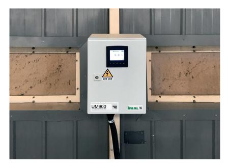
The UM900 microwave moisture meter owes its creation to the constant research and investigation into the development of new techniques to achieve accurate detection and monitoring of the parameters involved in the production process.
