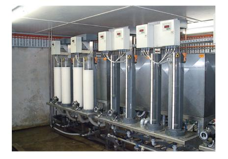
MULTIPUMP® is a component dosing system for fully automated chemical dosing operations. With the Multipump® dosing system, each chemical component of the glue mixture has its own dosing line, consisting of a motorized dosing pump, flow meter, and intermediate storage tank. This ensures precise and efficient dosing for optimal glue mixture consistency.
