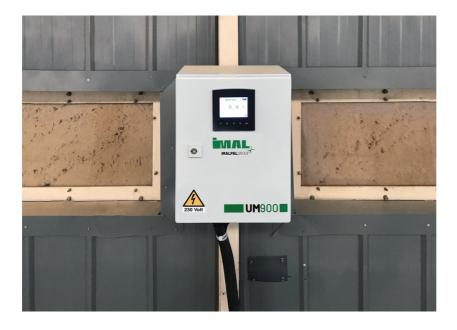
The UM900 is able to conduct the on-line measurement of the moisture content, density and temperature of the material analysed.
